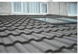
There was also workmanship issues with no roof flashings used and incorrect lapping with roof tiles.
